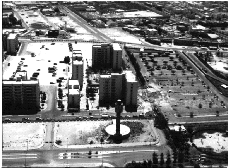
Figure J-5. Below, Photograph of Khobar Towers After the Bombing (Source: Report to the President and Congress on Protection of U.S. Forces Deployed Abroad (1996).)
